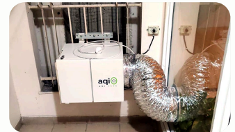
Bracketed to existing window bars
