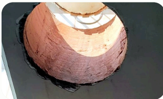
Through a wall with a clean core cut
